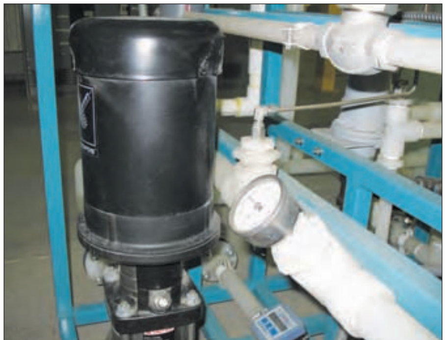
General purpose motors application examples (above and below). Both motors are general purpose with totally enclosed fan cooled enclosure designs and running at a constant RPM. These motors are servicing the exhaust system and pumps in water heating/cooling system while automation components such as valves, temperature sensors and controllers provide the appropriate automated control.
