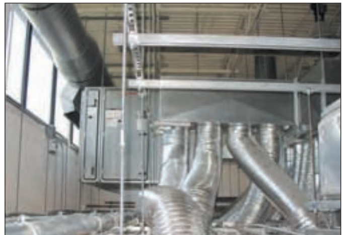
Inverter duty motor application example. The motor shown (above) is enclosed in the large air handling system (below). The motor and VFD control in this system is one of several motors driving and automatically adjusting multiple large forced air system with 14,000 CFM through hundreds of the HEPA filters, providing the appropriate amount of air changes, positive pressure and other environment controls to ensure the operational space contain no more than 10 particles of 0.5 microns in size.
